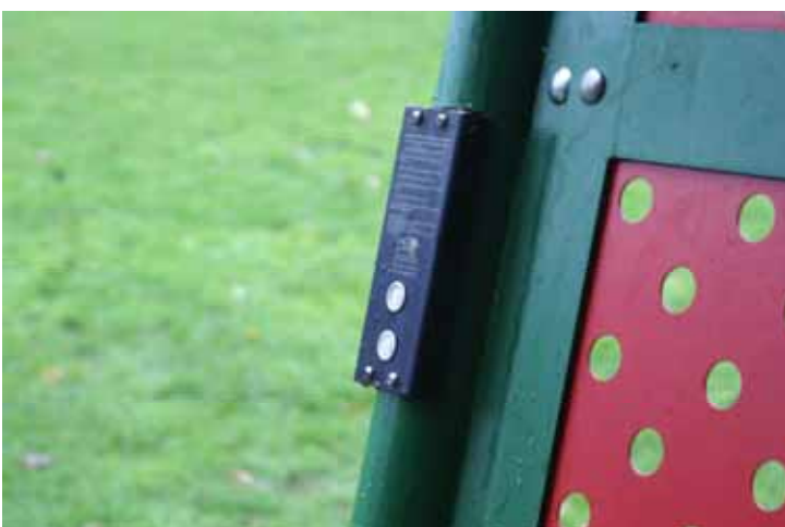
The audio/Bluetooth facilities in the shelter (speaker, receiver and on/off/channel buttons)– working and not vandalised.
