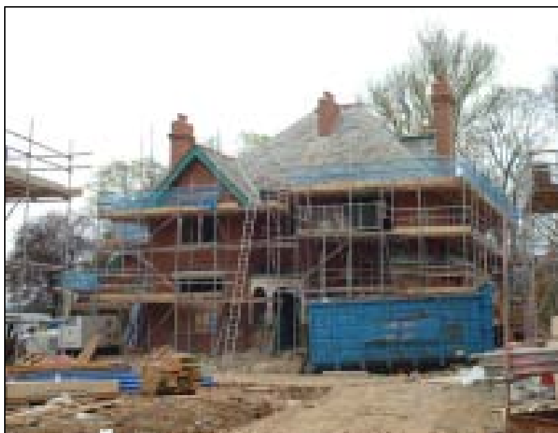
Conversion of former hospital building to affordable rented housing, Napsbury Park, London Colney.
