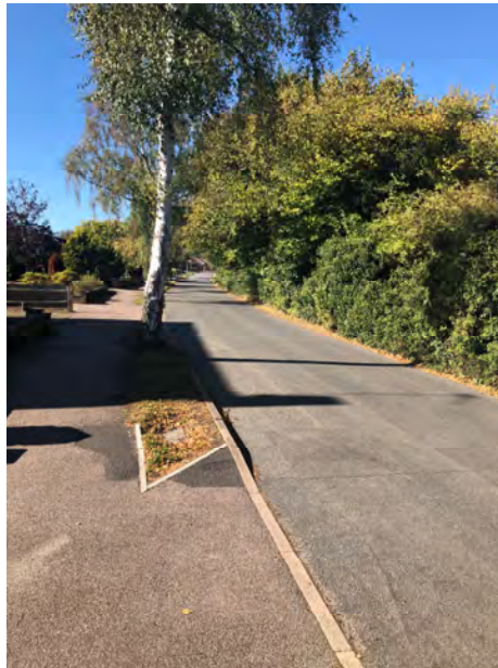
Photo 2 – Section of National Cycle Route 6 which runs parallel to Tippendell Lane
