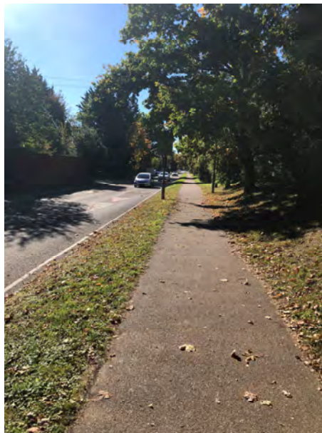
Photo 3 – Footway provision along Park Street Lane
