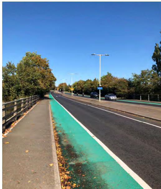
Photo 4 – Cycle lane provision along Watford Road Bridge
