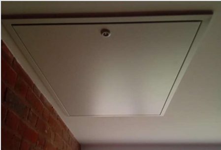
Upgraded – Communal ceiling, fire rated loft hatch, compartmentation in roof space
