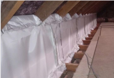
Upgraded – Communal ceiling, fire rated loft hatch, compartmentation in roof space
