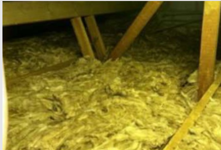
Loft Insulation – Upgraded
