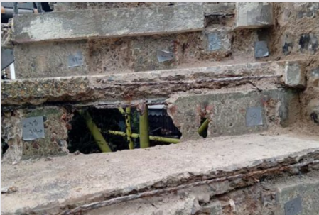
Structural Works – Including concrete repairs to stairs and balconies at Malthouse Court
