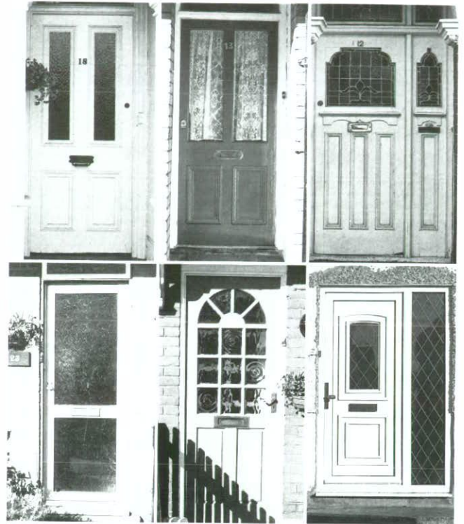
Original Victorian and Edwardian doors (top) and unsuitably-styled replacements (below).
