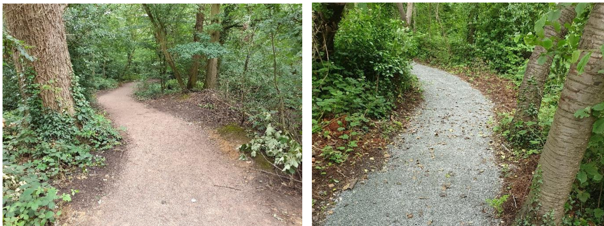
Figure 1. Examples of unbound crushed granite path surfacing that will be installed at Cunningham Field Open Space. The first photo is located at The Wick, St Albans. The second photo is from How Wood, St Albans.
