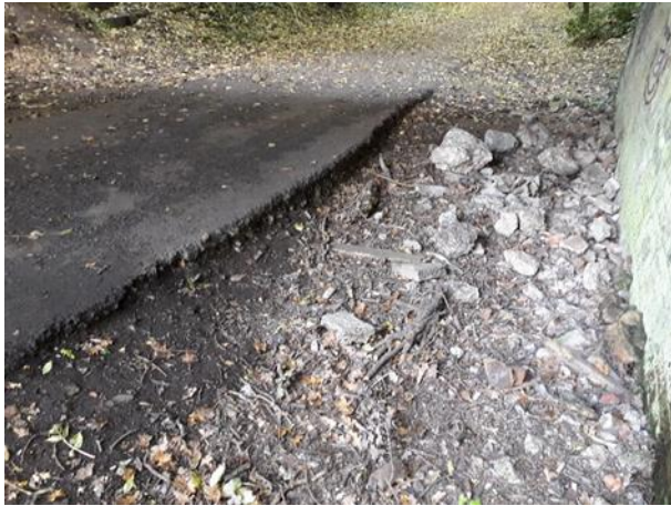
Eroded edge under Station Road bridge
