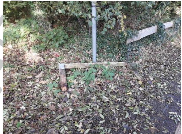
Damaged kickrail fencing
