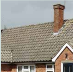
Roof of plain tile and chimney
