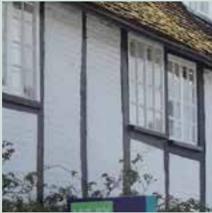
Mix of painted brick and timber
