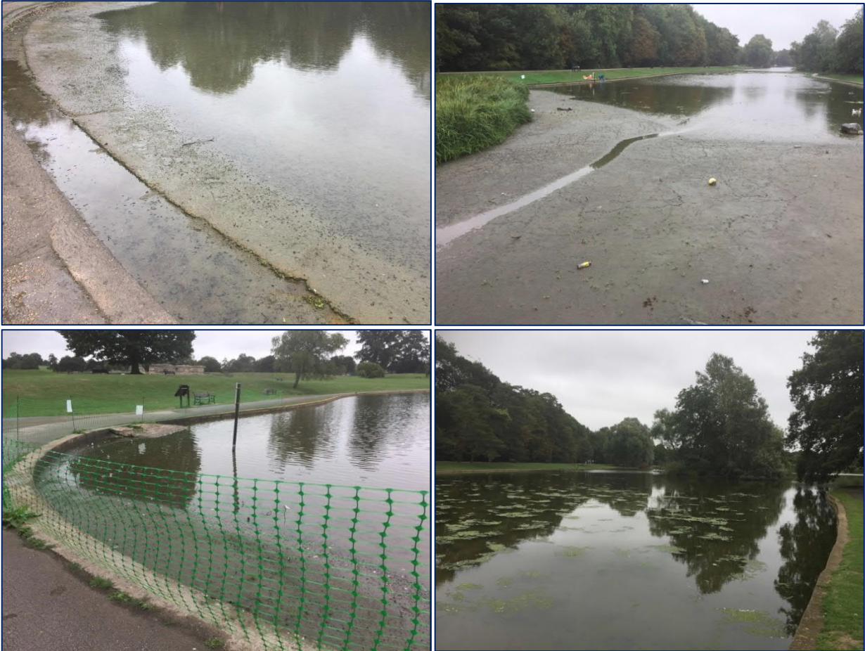
Plate 4.1 (top left) Concrete lake bed at the margins of the upper lake; Plate 4.2 (top right) Exposed sediment downstream of the weir between the upper and lower lake; Plate 4.3 (bottom left) Exposed sediment at the southwestern corner of the lower lake; Plate 4.4 (bottom right) Algal accumulations on the surface of the lower lake
