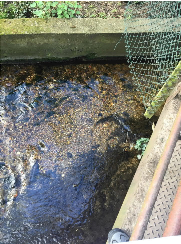
Plate 3.19 Local channel narrowing created by woody feature exposing gravel bed
