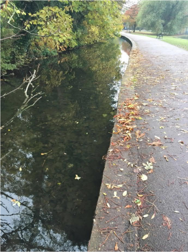
Plate 3.9 Fine sediment deposition, lateral berms and concrete lined right bank
