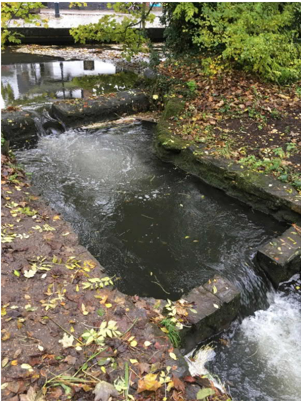
Plate 3.28. Upstream extent of the fish pass structure in Reach 1
