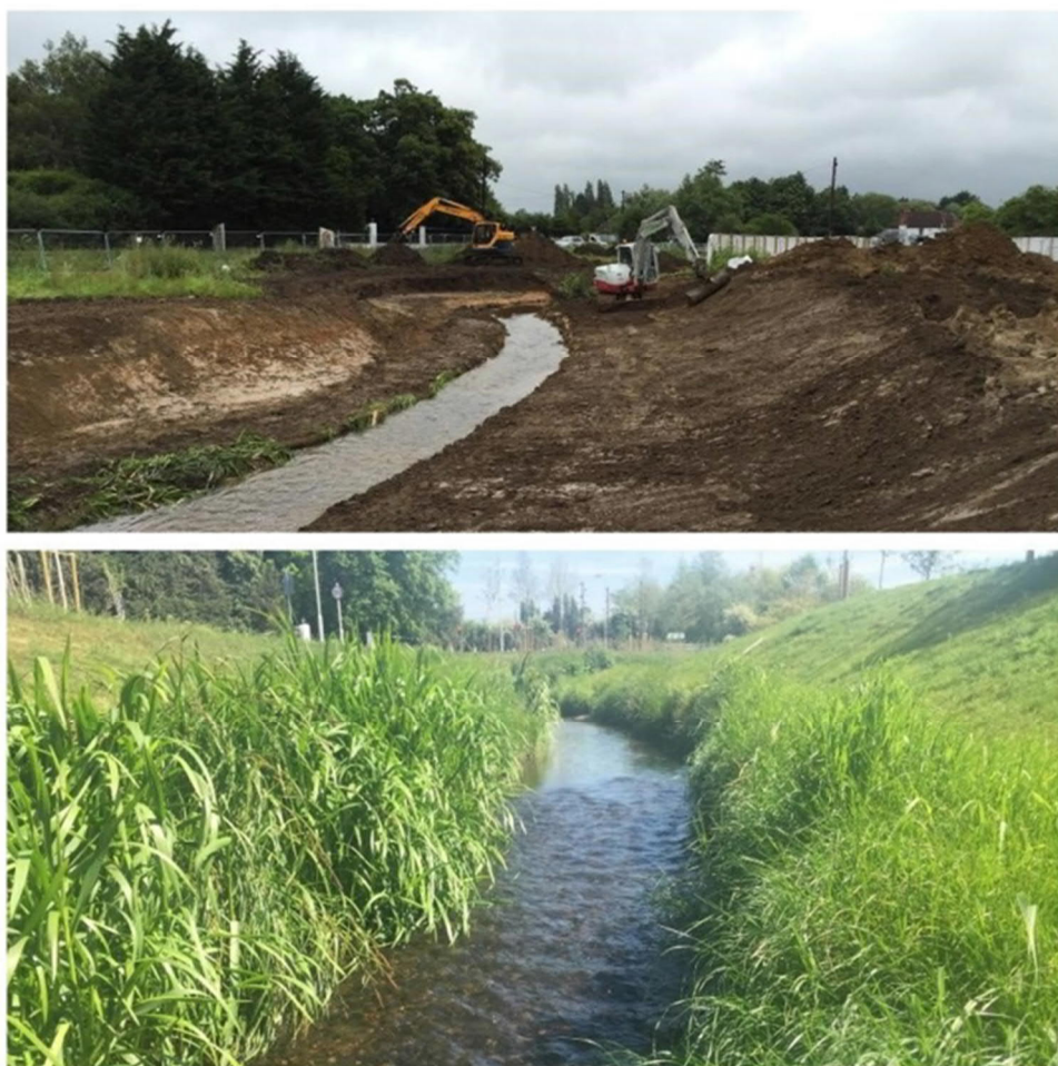
Plate 4.5 An established section of restored river channel on the River Bulbourne, Hertfordshire, with vegetated berms developing in the margins (Photo courtesy of Five Rivers Ltd)
