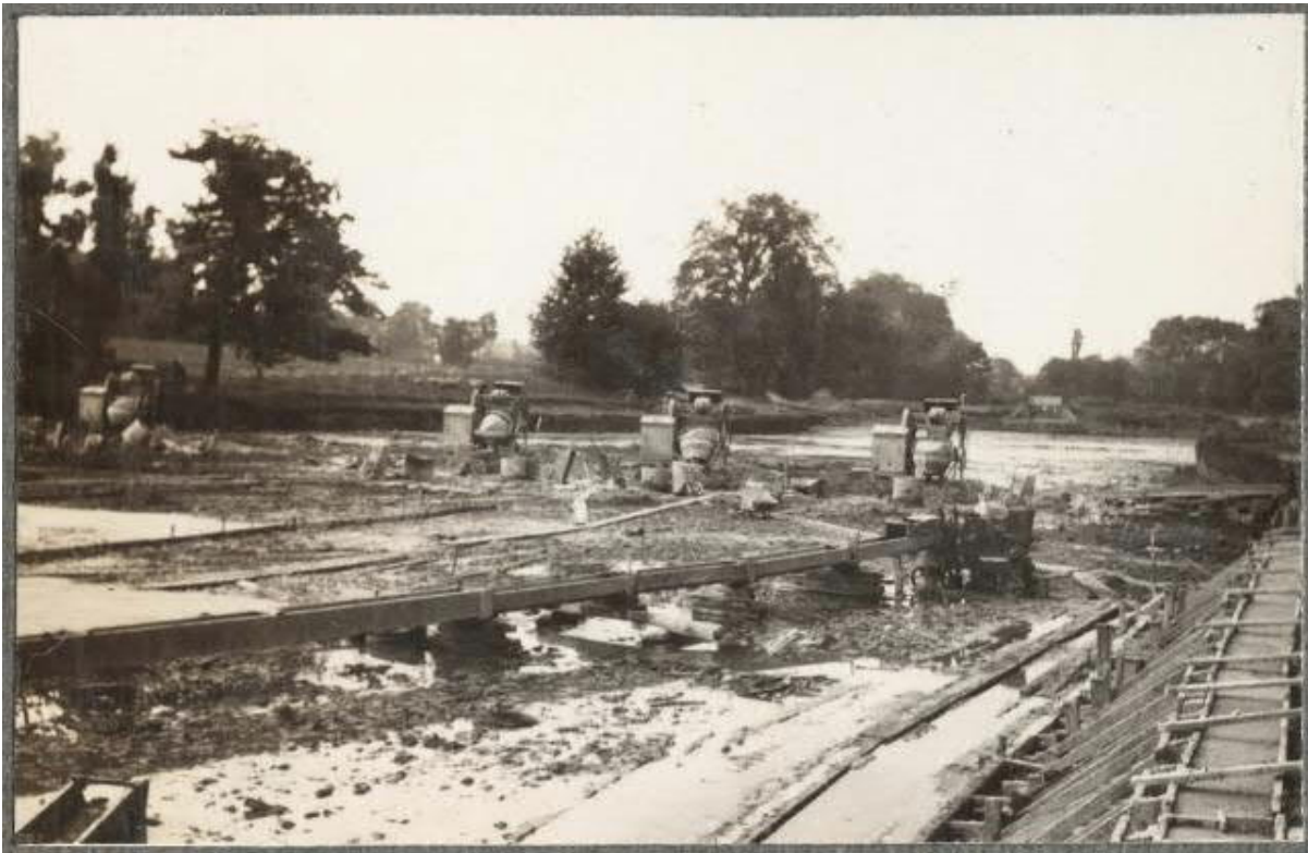
Plate 4.1 – shows the concrete base of the lake under construction
