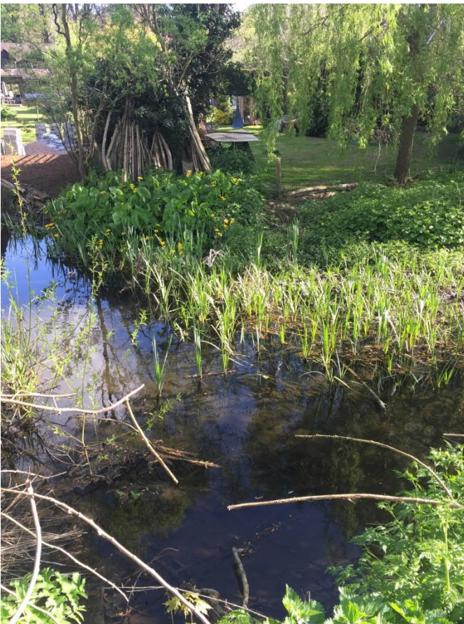
Plate 3.15 Vegetated fine sediment lateral berm
