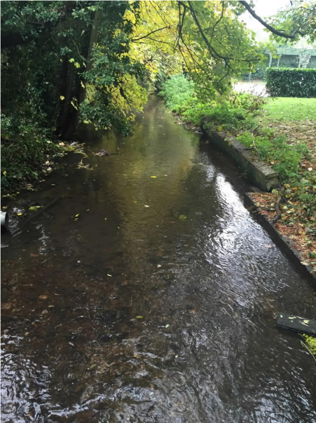
Plate 3.17 Failing right bank hard protection and low energy glide flow type throughout Reach 3
