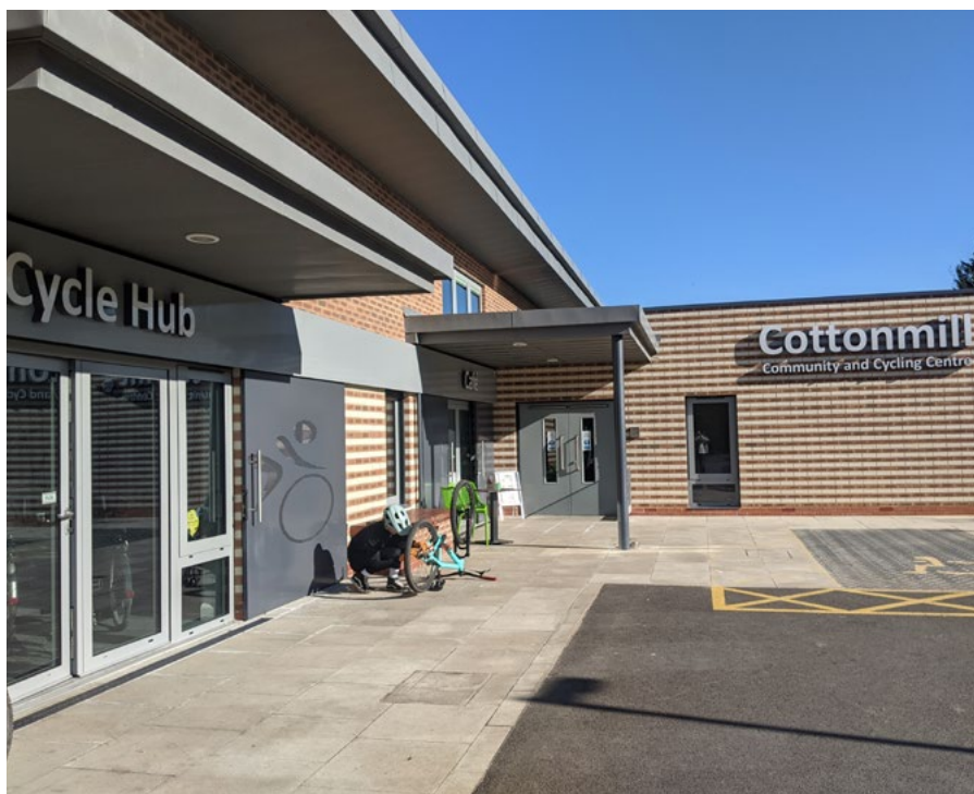
Cottonmill Community and Cycling Centre, St Albans. Completed 2022.
