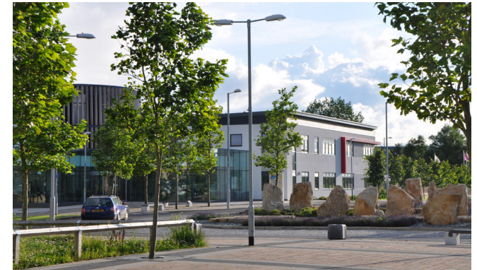
The Enterprise Centre in Priors Hall, Corby
