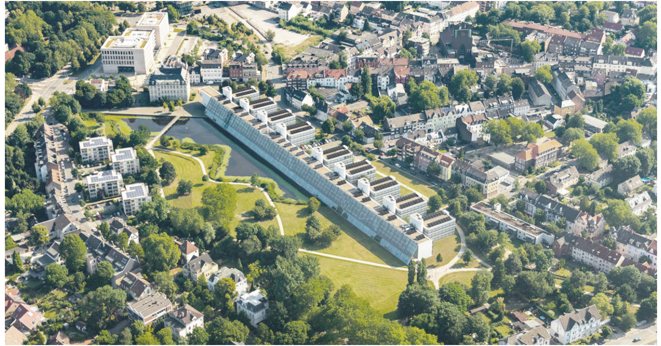
Tilted and interactive glass façade at the Gelsenkirchen Science Park, with PV Solar Plant on the Roof
