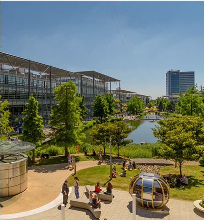
Solar shading at Chiswick Park
