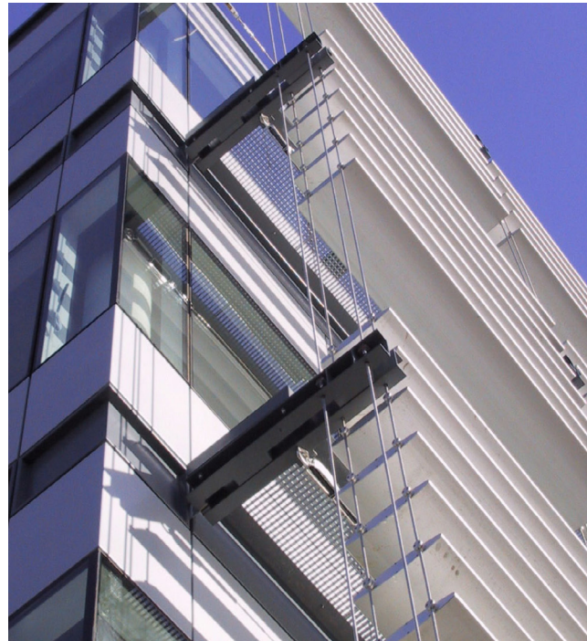
Horizontal louvres at 300 Longwater Avenue
