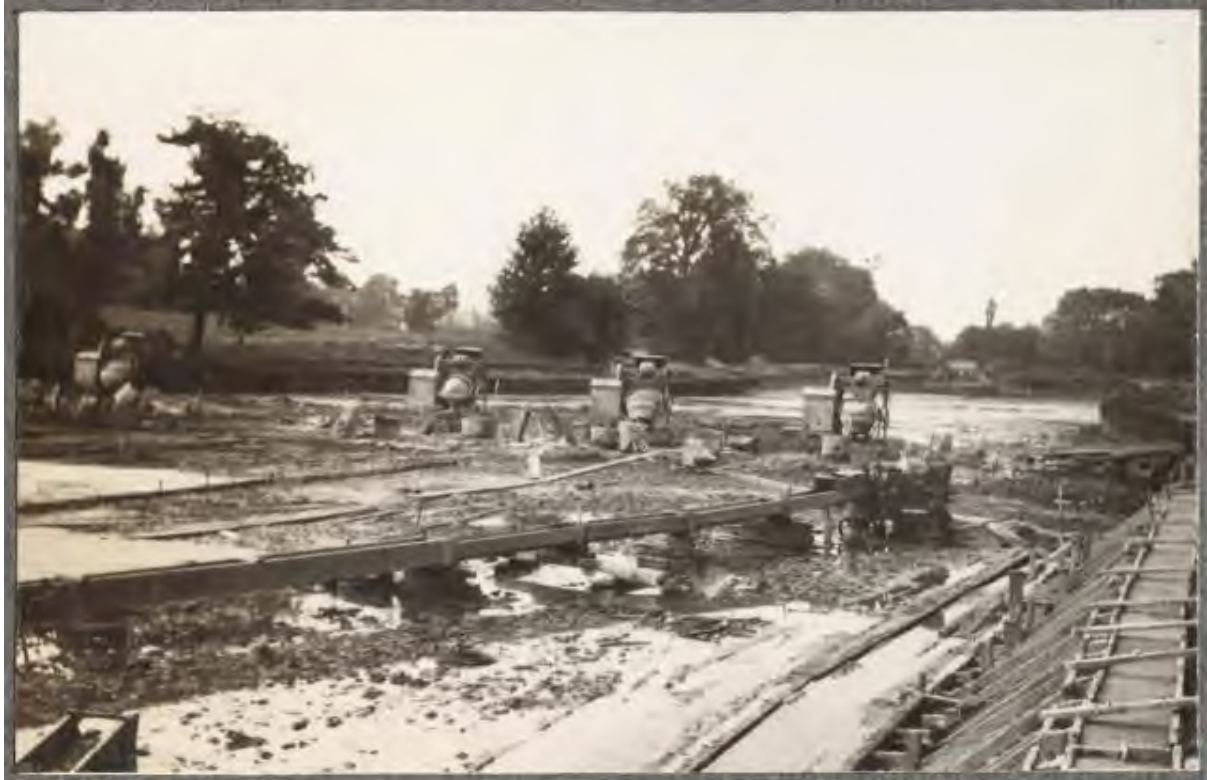
Figure 4 – shows the concrete base of the lake under construction
