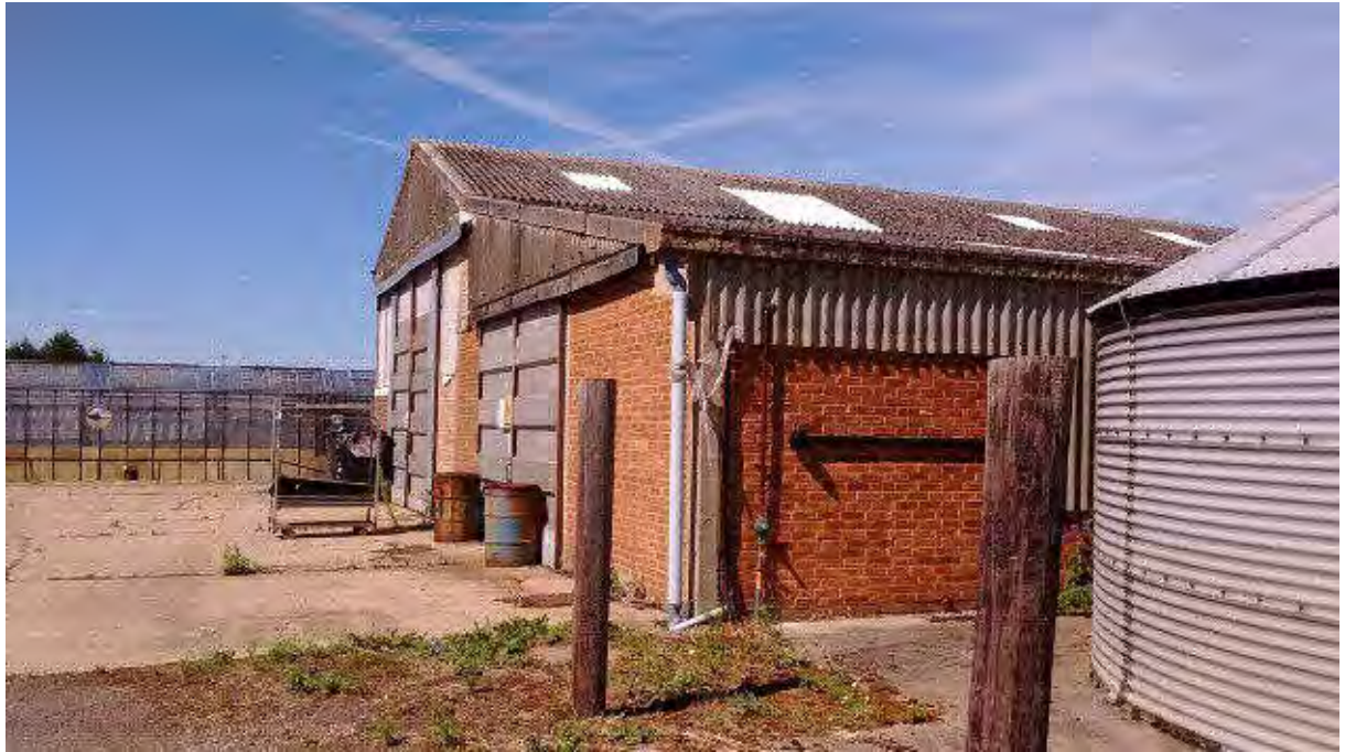
Photograph 9: Potential ACM was noted within the roofing and wall materials of a building located in the north-western site corner, facing west.
