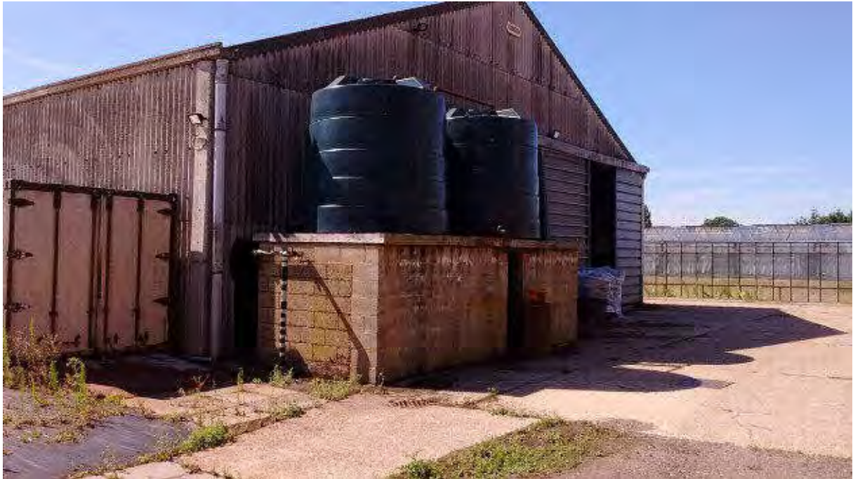
Photograph 13: Two ASTs were noted in the western site area. Potential ACM was noted within the roofing and wall materials of a building located adjacent to the ASTs, facing south-west.
