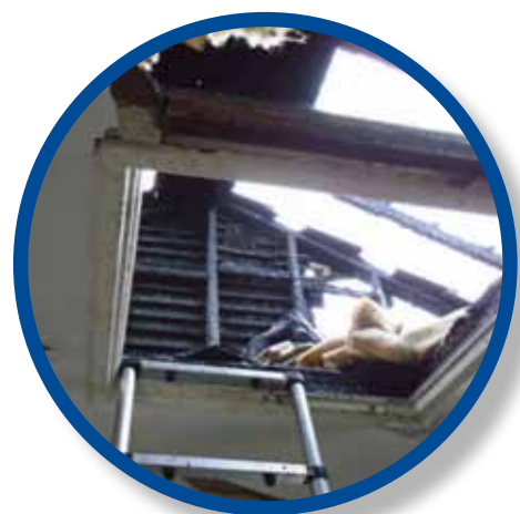
Unauthorised loft works caused severe fire damage to this property.
