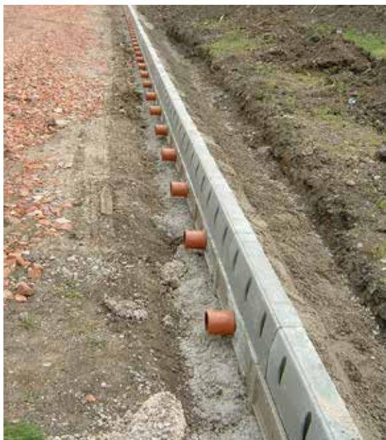
Figure 20.8 Macro pervious pavement under construction in the Midlands – kerb drain collector/ pollution trap with connectors before placing diffusers and permeable sub-base to left (courtesy Phil Tomlinson)
