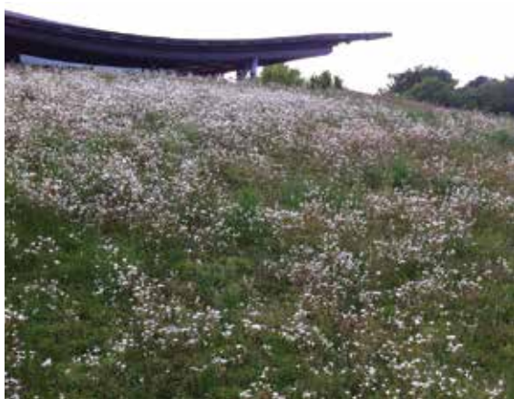
Figure 12.2 The Savill Garden extensive green roof
