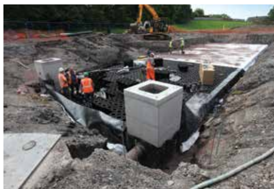
Figure 21.5 Man access chambers located within the structure (courtesy Aco Limited)
