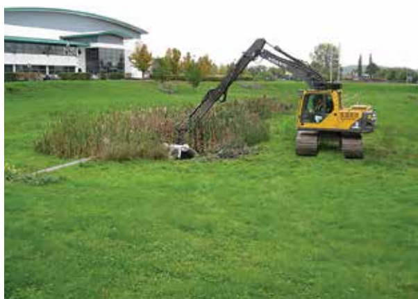
Figure 32.2 De-silting (courtesy Bedford Group of Drainage Boards)
