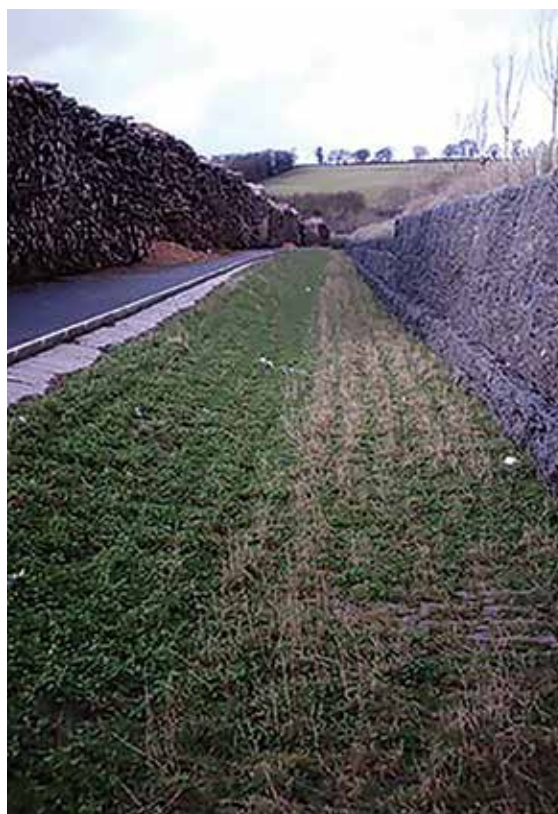
Figure 17.6 Swale with vertical side (courtesy EPG Limited)
