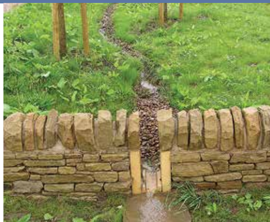
Figure 6.2 Conveyance component (courtesy Sheffield City Council)
