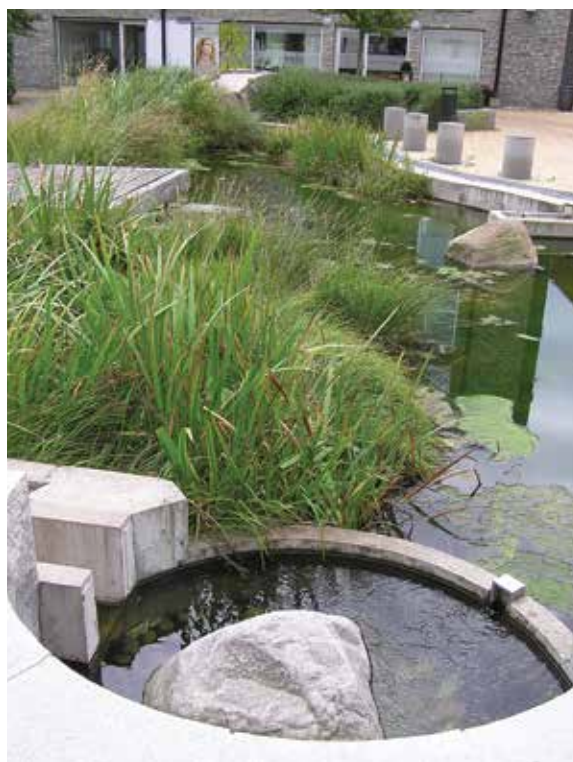
Figure 23.7 Pond with baffles and islands, Augustenborg, Sweden
