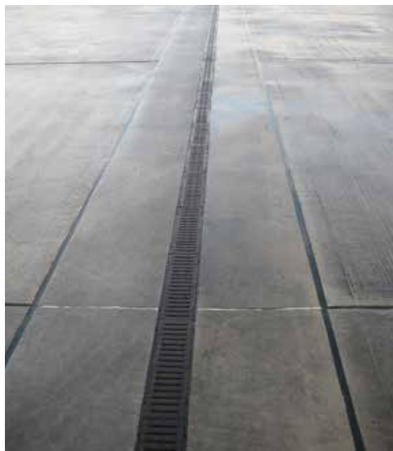
Figure 20.9 Macro pervious pavement in warehouse yard in north-west England with channel collection/ pollution trap and concrete pavement construction (courtesy EPG Limited)
