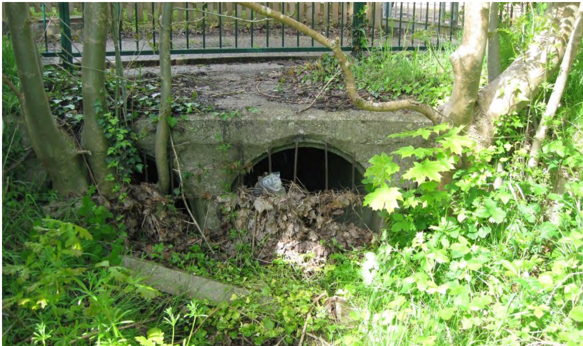
Photograph 5: Unmaintained culverts blocked by trees, plants & debris
