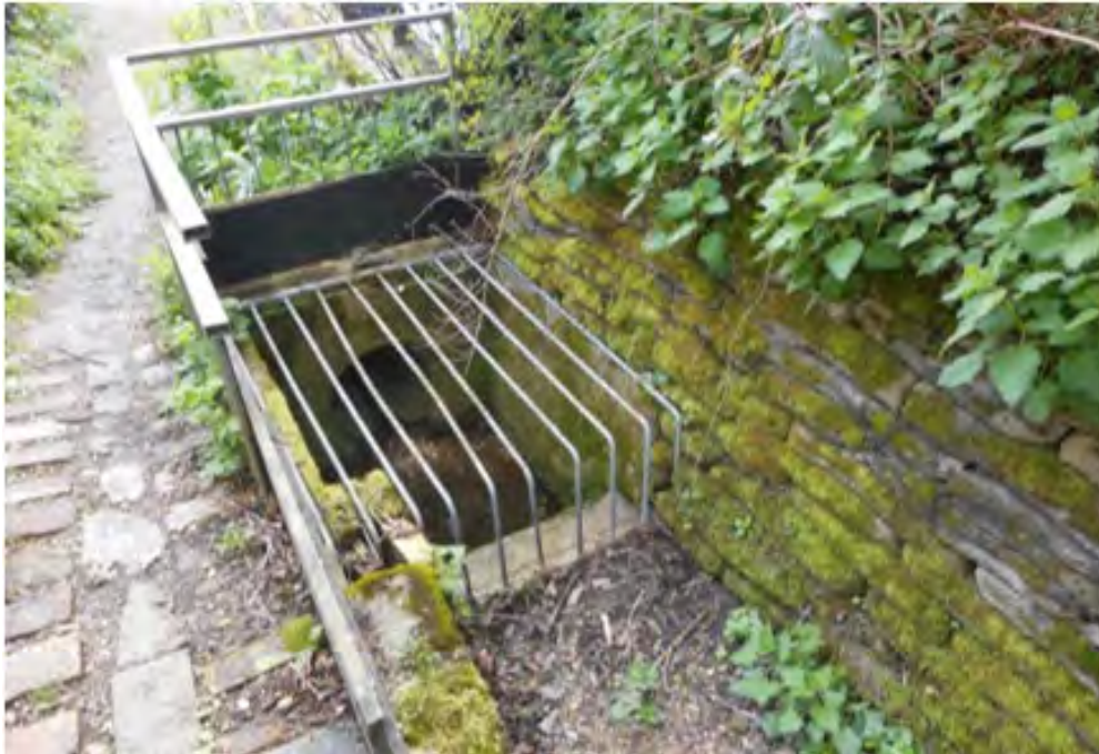
Photograph 6: A culvert on a small watercourse
