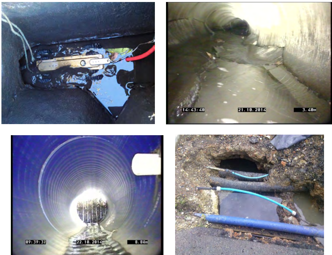
Photograph 16: Investigations and CCTV surveys of culverts
