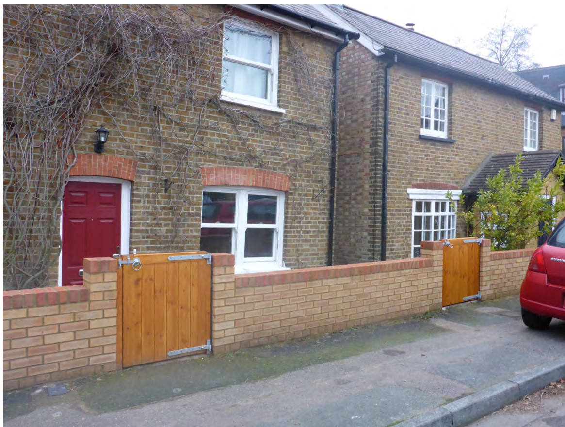
Photograph 18: Boundary wall and flood gates
