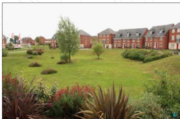
Infiltration / Attenuation Basin
