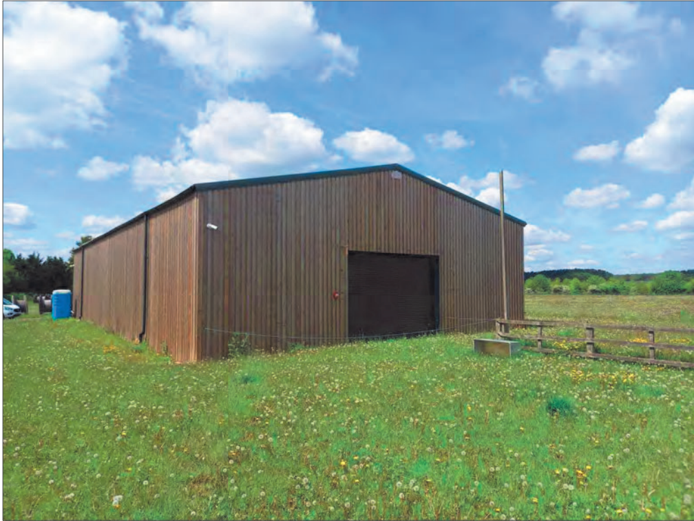
Hay storage building
