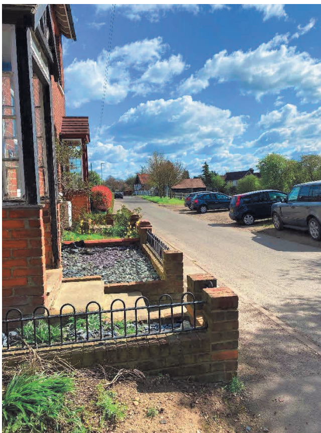
Figure 2 View of Footway Infrastructure along Chiswell Green Lane
