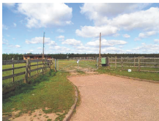
Figure 16 View of Secondary Access off The Croft
