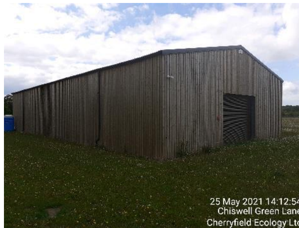
Figure 4: Rear and side elevations of B1.
