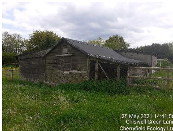
Figure 8: Rear and side elevations of B2.
