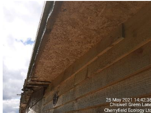
Figure 20: Example of tight-fitting overhanging eaves.
