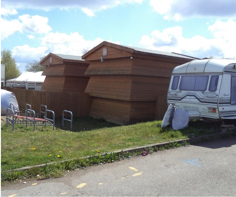
Photo A: Photo of Beehive toilet block, as seen on site 5 May 2021
