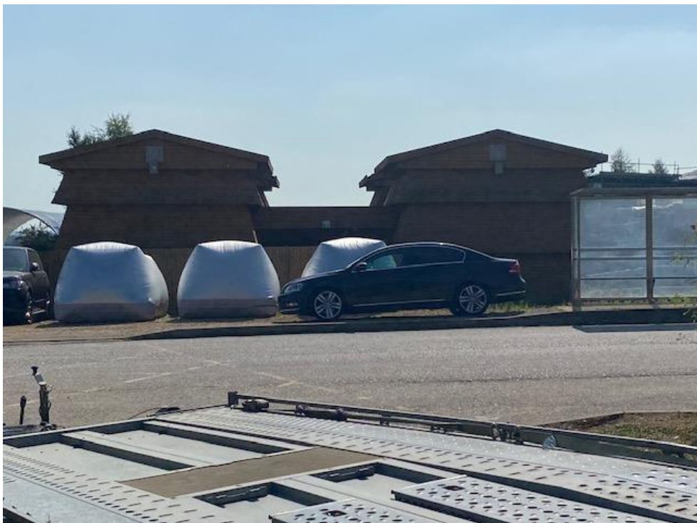
07 September 2021 – Site visit photo of 'A' – toilet block.
