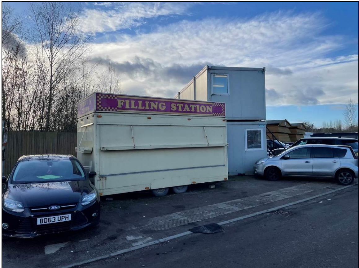
Photograph F – Showing some of the current structures on the site.
