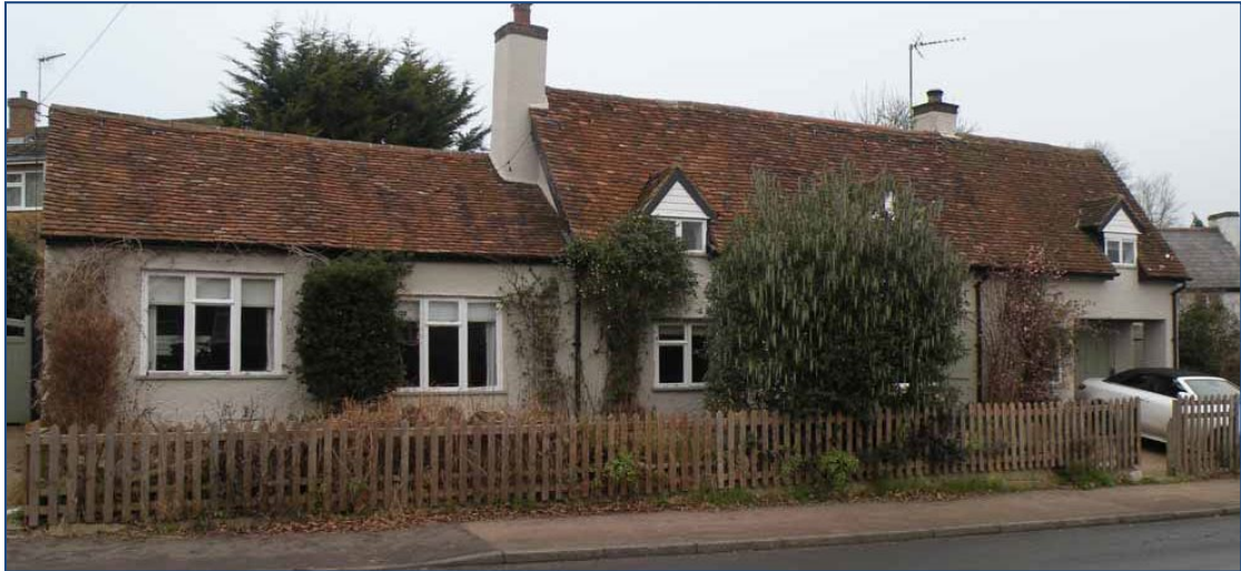
Figure 22 No.94 High Street, from High Street
