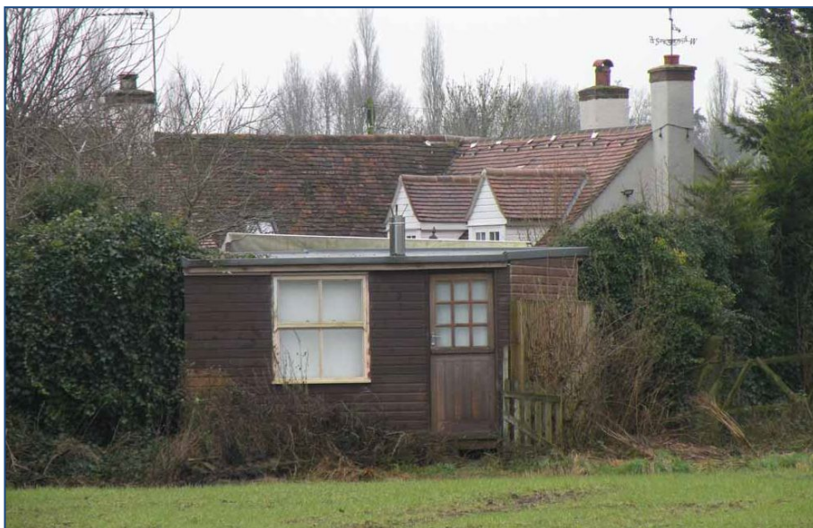
Figure 27 No.94 High Street rear elevation from SE corner of PDA, showing attic windows and shed on PDA boundary
