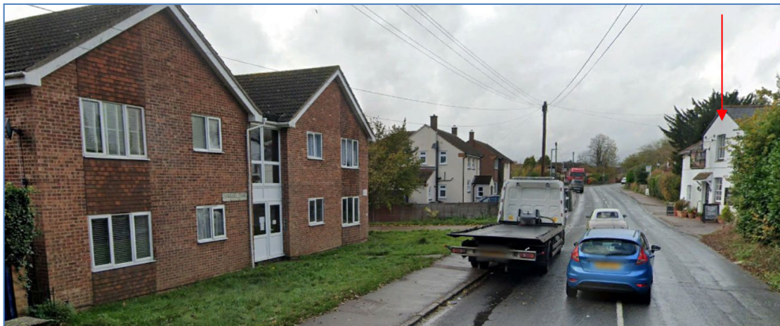
Figure 14 Looking west along High Street with Crooked Billet PH (arrowed) (© Google, base photo)
