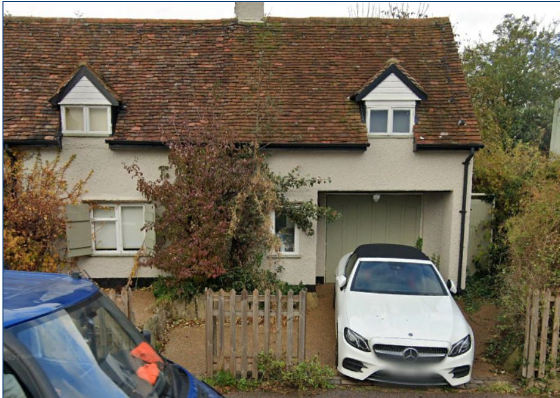
Figure 23 No.94 High Street, showing garage in eastern extension (© Google)
