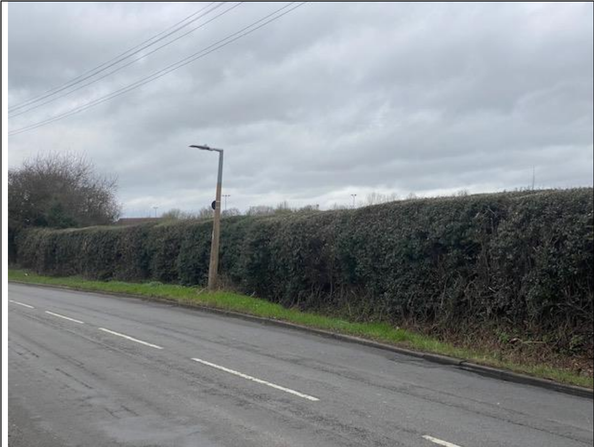
5 Above from pavement outside 53 High St
