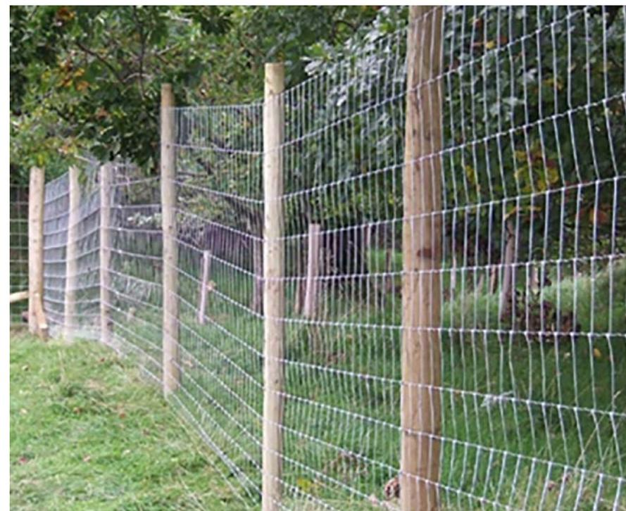
**3.4** Deer fencing, which should be 1.8m high, is most successful where it is installed in combination with the construction of 'green bridges' and under / over passes, whereby the fencing channels the animals to the safe crossing points.
