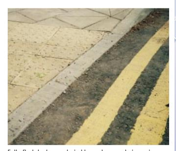
Fully flush kerbs are desirable, so long as drainage is adequate. *Courtesy: Tony Russell.*
