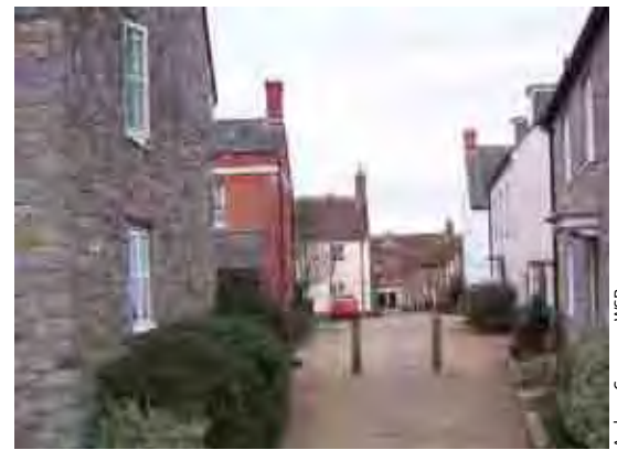
Figure 4.9 A good example of a pedestrian/cycle route at Poundbury, Dorchester. It is short, direct and with good surveillance.
