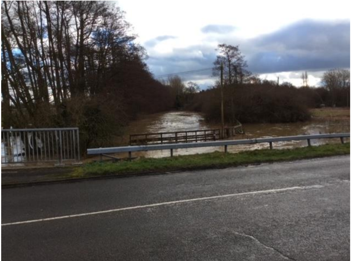
Taken 20 th February 2014 from Coursers Road bridge Colney Heath
