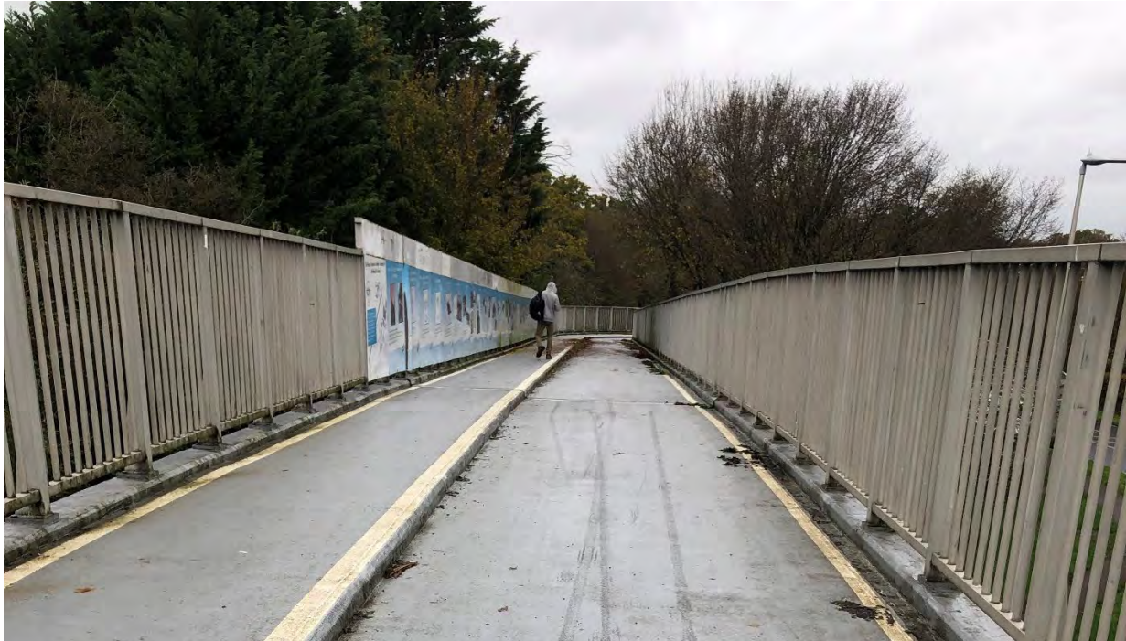
Fig 13 – South Way Overbridge
