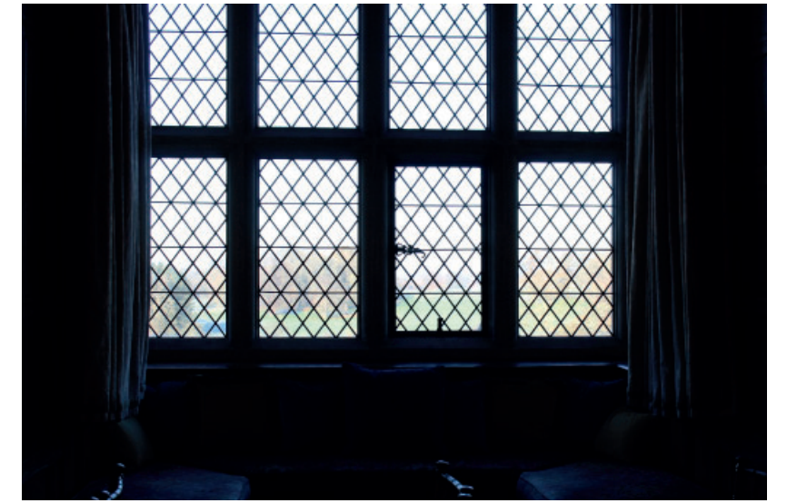
View of the window from the interior
