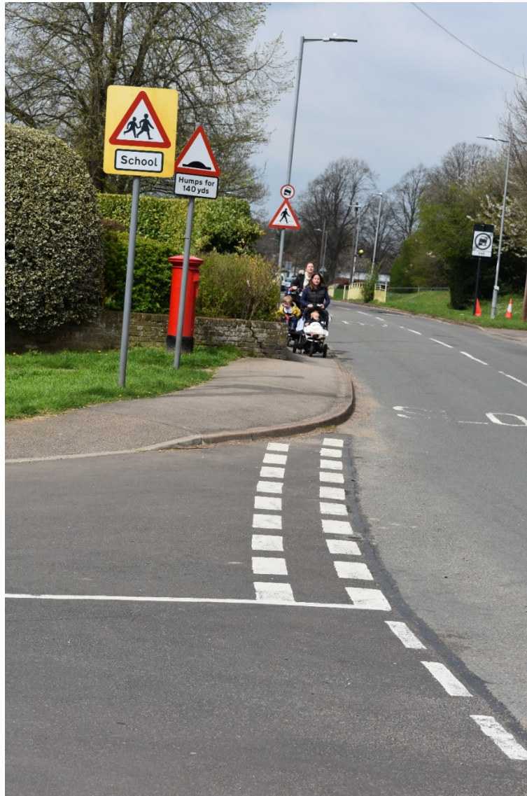
Junction of High Street and Park Lane – an example of the problem due to the width of the pavement
