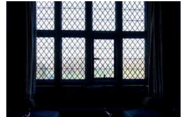
View of the window from the interior
