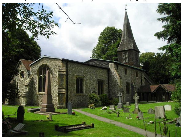
The spire of St Stephen's is a Victorian addition but the church has retained the traditional materials of flint and stone.
