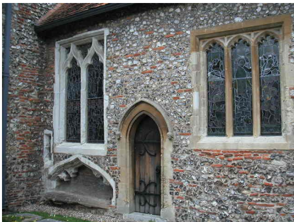
The external elevations of the building display reused materials, such as Roman bricks and carved stone features.
