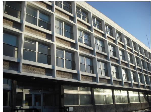
Concrete framing on Beaver House.
