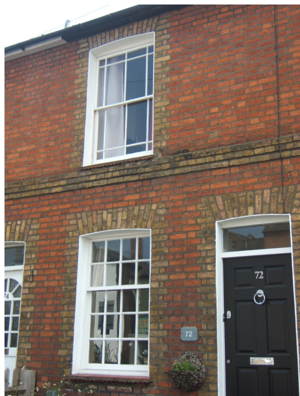
A house in Lattimore Road displaying red brick with yellow brick detailing and a sash window with margin lights.
