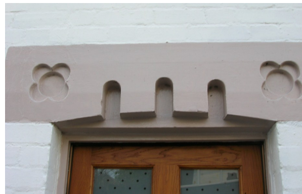
Riverside Road terraces have stone headers with moulded patterns.
