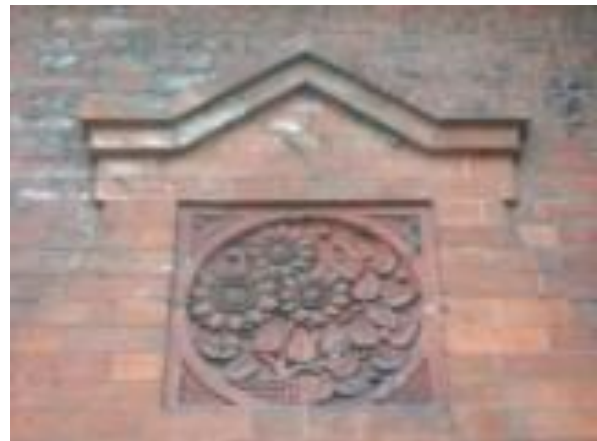
The detailing and range of materials used, such as terracotta decorative panels, demonstrate the craft skills of C19.
