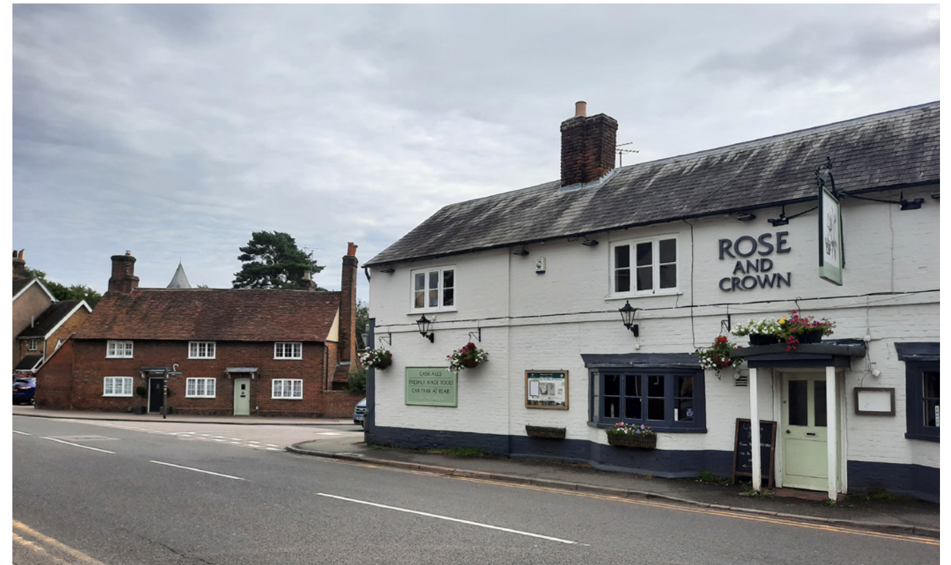
The Rose and Crown dates to at least the C16. Both the PH and 20-22 High Street are timber framed, with later brick façades
