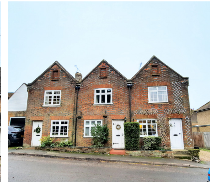
4-6 Church End is grade II listed, the rear range is thought to date to the C16-17
