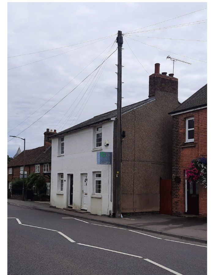
Nos. 40-42 High Street, formerly the White Horse PH, the beer cellar hatches are still evident
