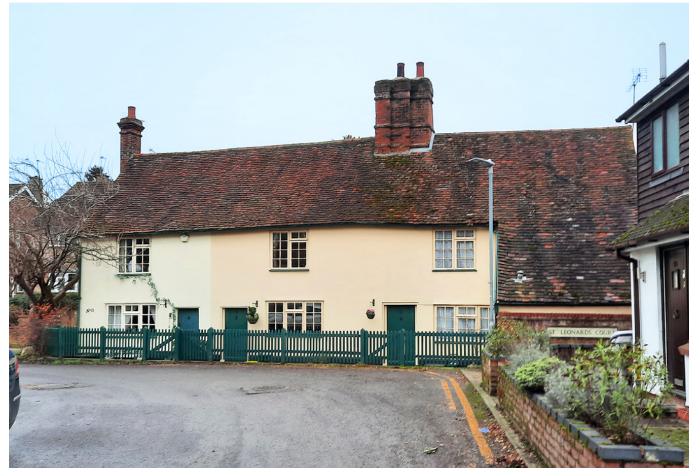
9-11 Church End is grade II listed and has C17 features, including the large red brick chimney stack of joined square shafts
