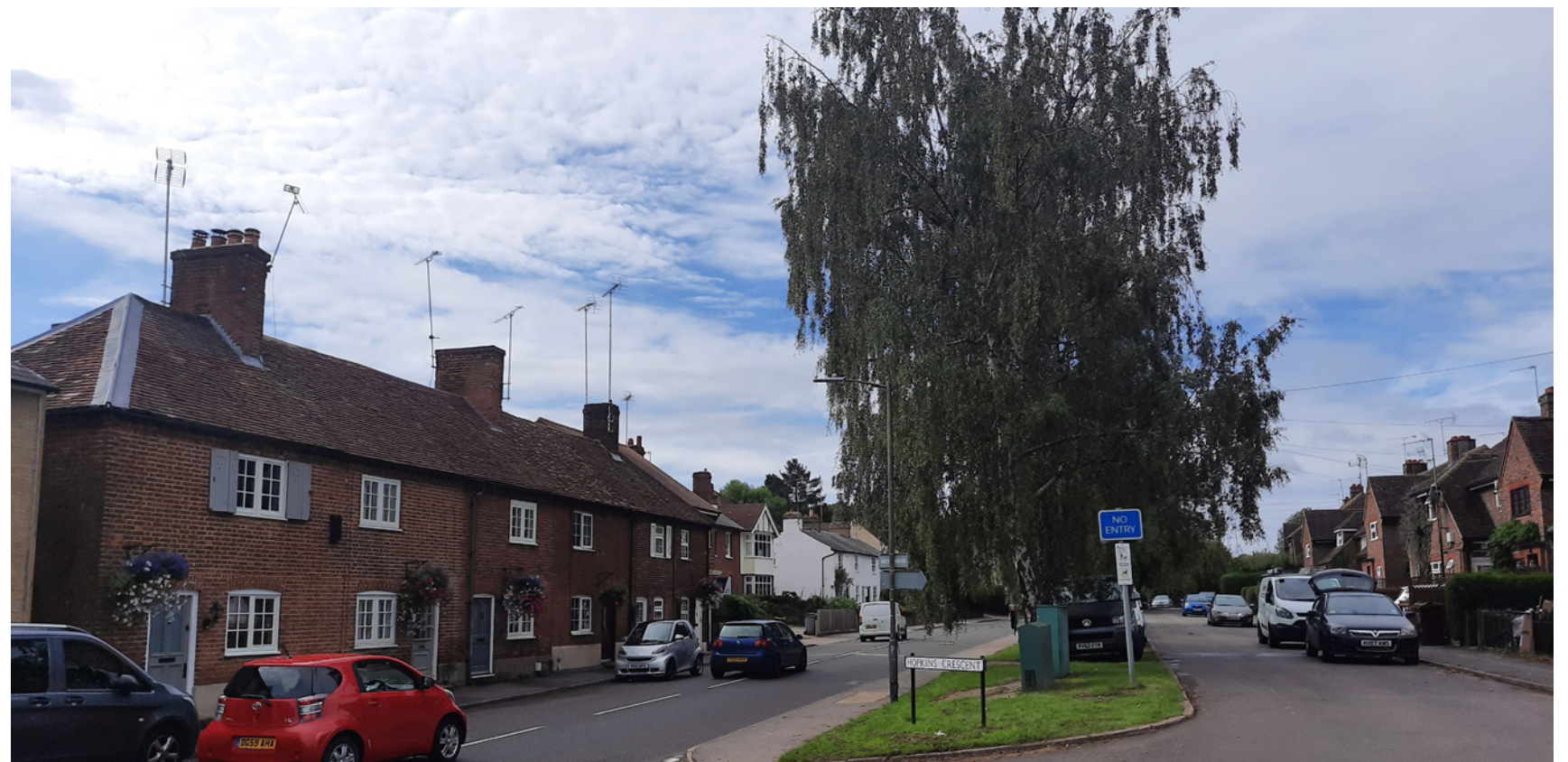
The south side of the High Street displays the key characteristics of the conservation area, including the close relationship of the buildings between each other and the street and the typical materials and building form.
