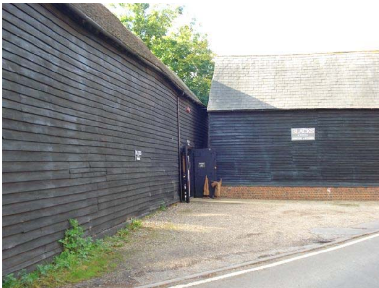
Barn to south of New Barnes Mill
