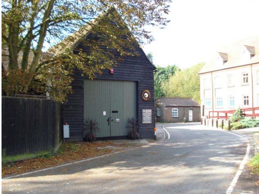
Barn to south of New Barnes Mill
