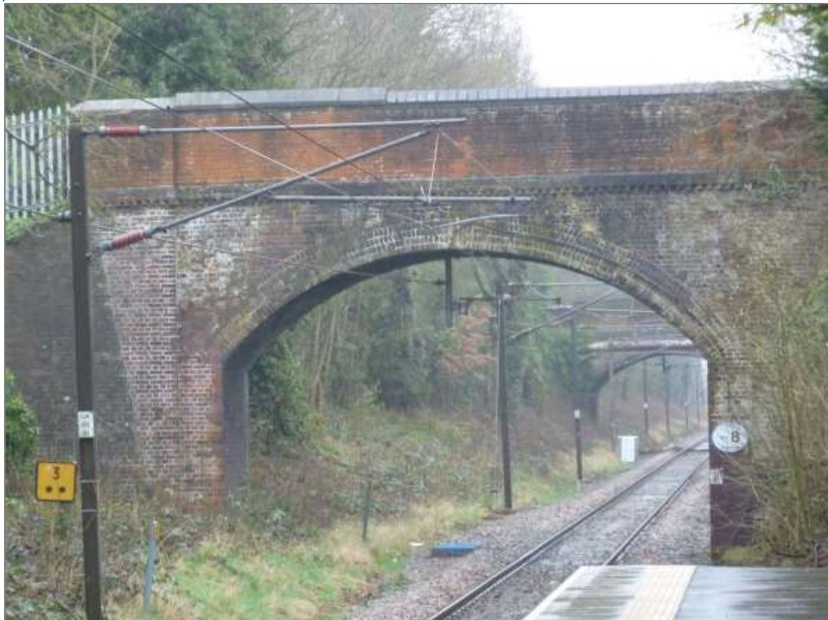
FIGURE 11: MASONRY ARCH FOOTBRIDGE TO THE NORTH OF BRICKET WOOD STATION
