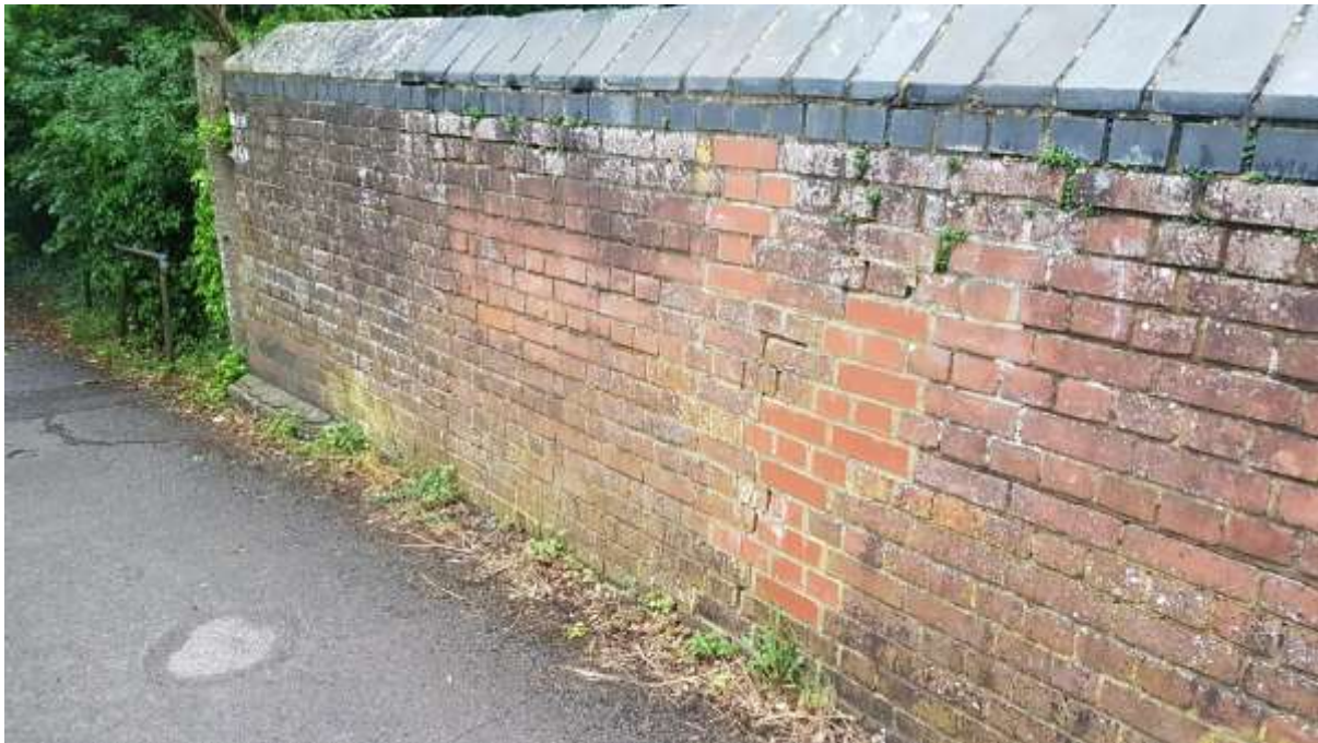
FIGURE 12: EXAMPLE FRACTURE TO PARAPET AT NORTH WEST OF THE BRIDGE (ADJACENT TO PREVIOUS REPAIR)
