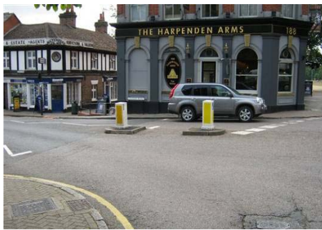
Plate 5 - Splitter island with no dropped kerbs in the bell mouth of Station Road
