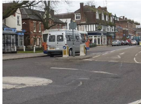
Plate 6 - Splitter island without pedestrian facilities to the north of the mini roundabout junction with Station Road.
