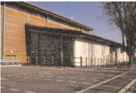
Galvanised steel columns and cedarboard cladding contribute to this interesting, low maintenance sports centre exterior.
