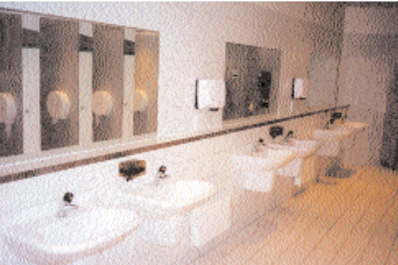
Basin ducts protect pipework and simplify surface cleaning. In this example ‘between basin’ dispensers help conceal any soap spillage.
